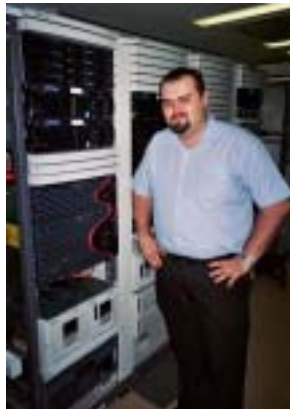
Marcus Armour, System Administrator, Tweed Shire Council with 9200 SAN
